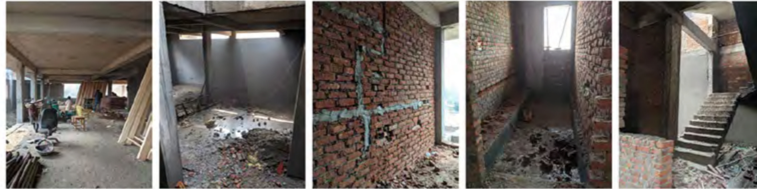
The entry stilt level used for parking; the area on the left will be covered with a jali to ensure privacy, while keeping the area ventilated The basement level double height seen through the cut out. It is primarily lit by clear stories Conduits places in wall before it is plastered Sunken Slab for toilets with a ventilation window at the farther end. The Staircase next to the cut out and the elevator
